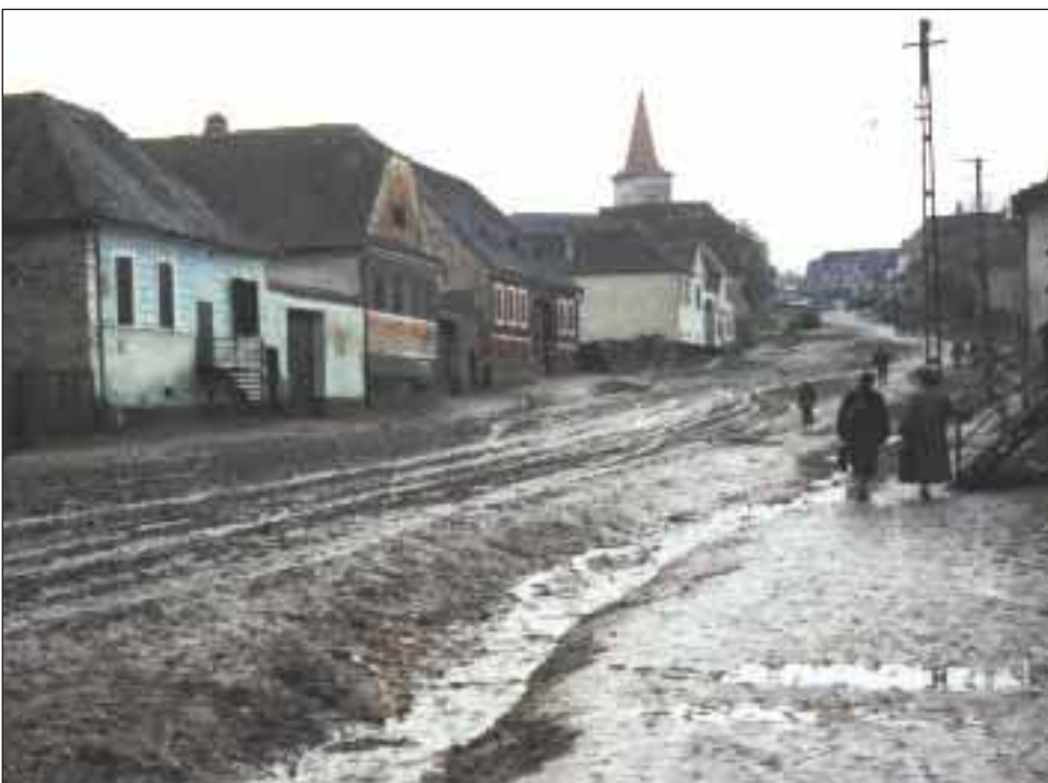
28th April 1999 - the church is derelict
